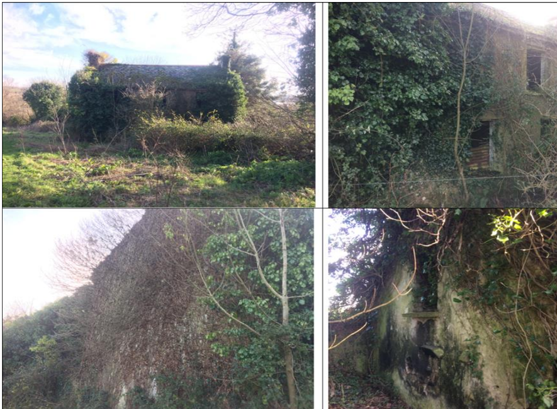
Photographs 1 – 4: External elevations of the former dwelling
